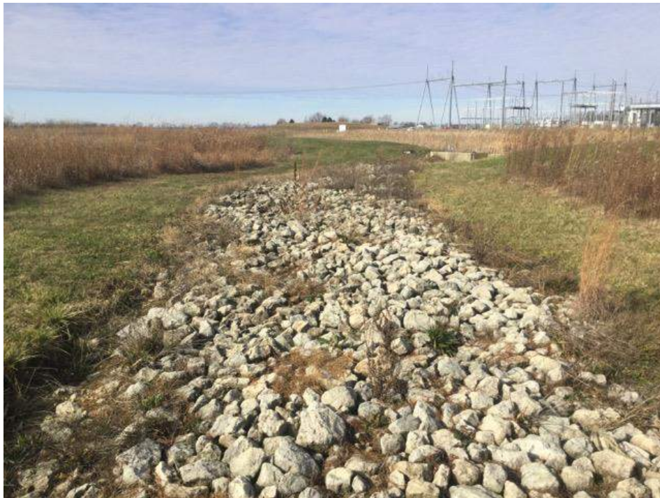
Photo Location 5. View of rock channel outlet. Photograph taken facing northwest.
