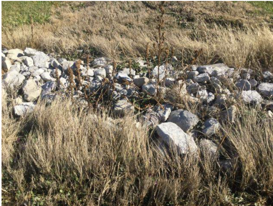
Photo Location 6. View of rock check dam.
